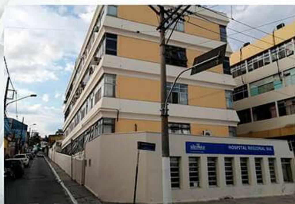
HOSPITAL REGIONAL SUL
