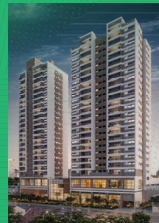
Club Station - Penha Rua Doutor Suzano Brandão, 720 Penha
